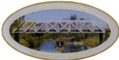
WW 0004 18 District 201 N1 (AUS) The Bendmeer Bridge NSW
